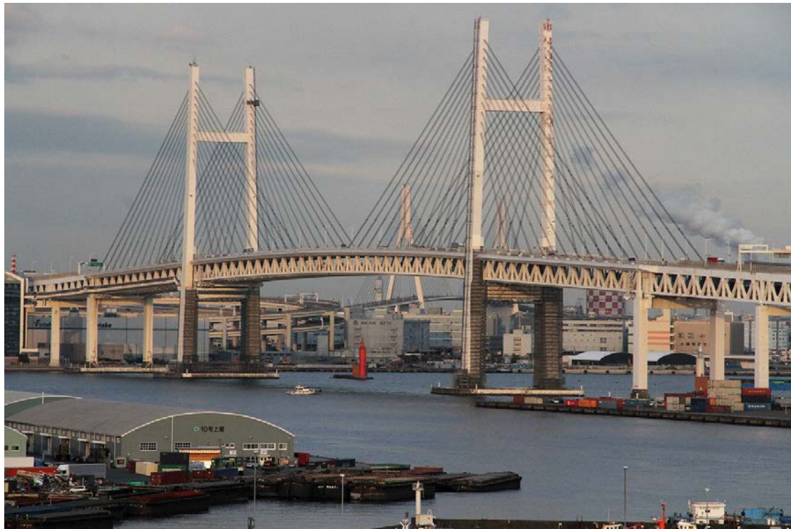
Yokohama Bay Bridge
